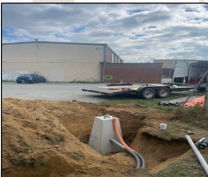
Civil engineers install conduits into light standard.
